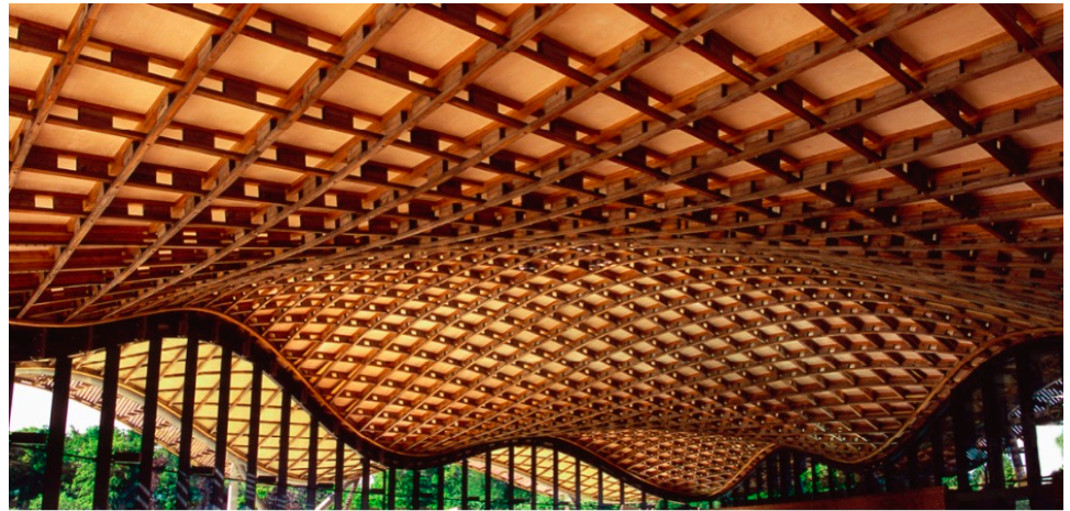
Figure A.7: Roof of the Savill Building
