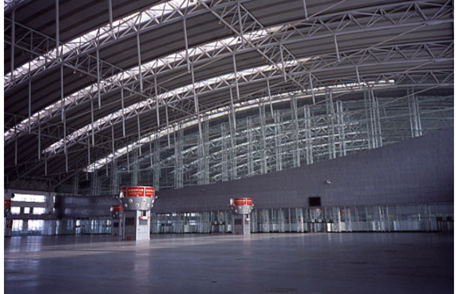
From: http://aloss.biz/en/8958 (Harbin Gymnasium - 2004 Shizhao Shen, Feng Fan et al, Structural engineers)
