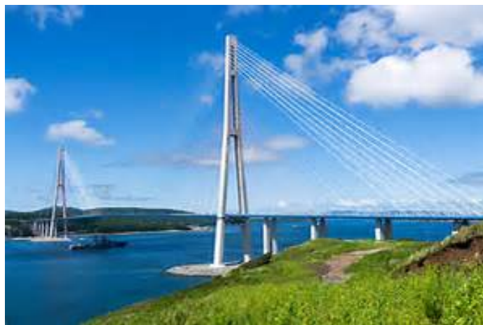
Figure 2. Bridge over the Eastern Bosphorus strait in Vladivostok (60 + 72 + 84 + 3 × 1104 × 3 + 84 + 72 + 60 m)
