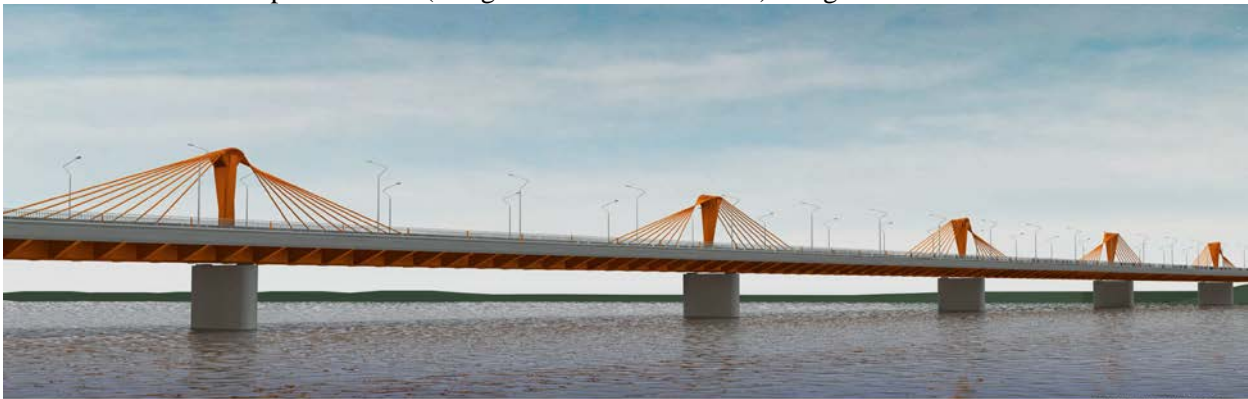
Figure 1 Bridge over the Daugava river in Riga (49,5 + 77,0 + 5×111,0 + 77,0 + 49,5 m.)
