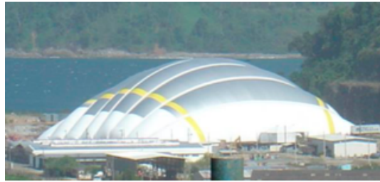
Figure 3: (a) A large pneumatic dome reinforced by sliding cables; (b) finite element mesh and equilibrium geometry under internal pressure.
